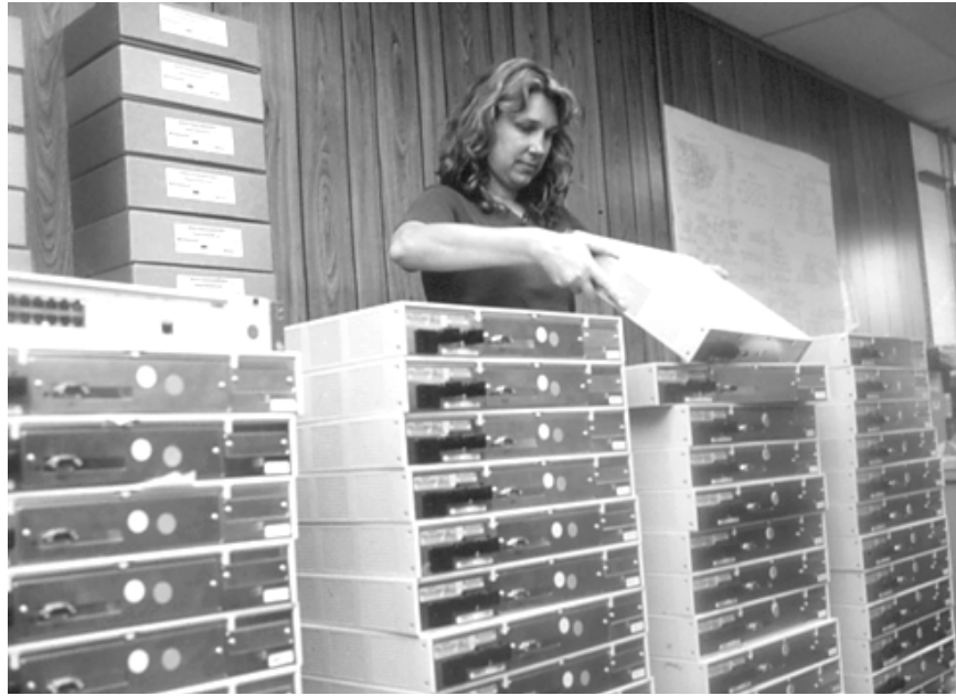
Alice Harrison inspects one of the more than 600 link switches to be installed this summer.
